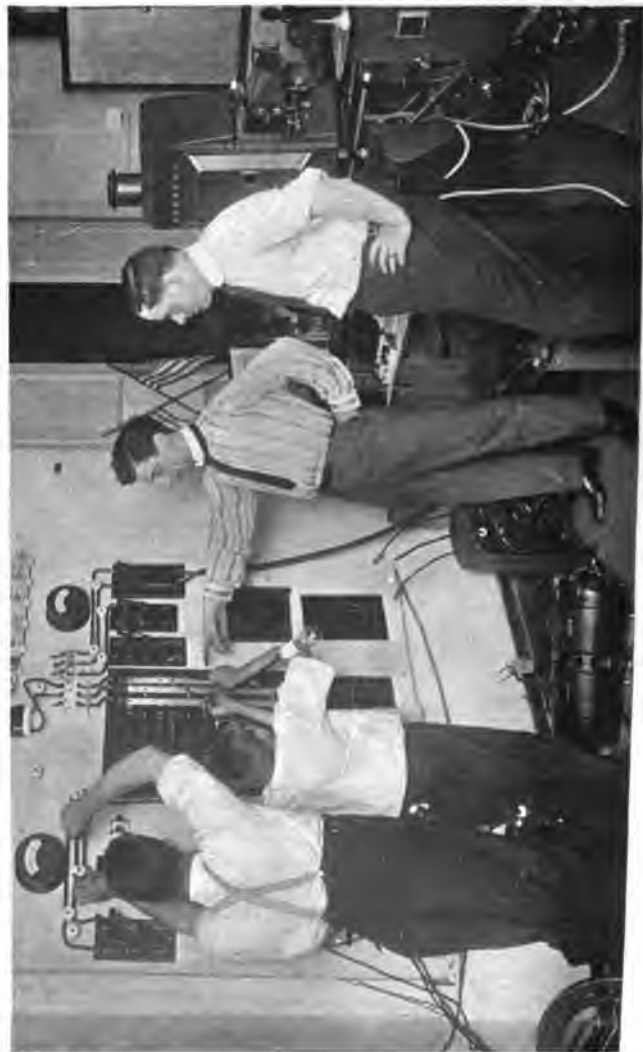
Installing electric wiring system at Red Cross Institute
